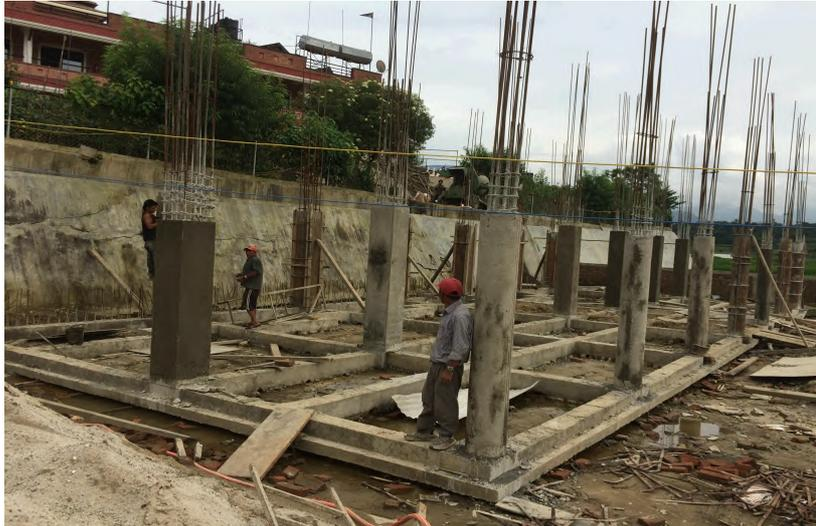
On the 13<sup>th</sup> the tie beams for the ground level was cast in concrete and shortly after the casting of pillars began and is being completed.
